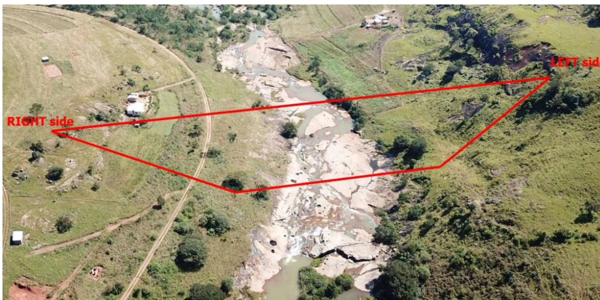
Figure 5-5: Aerial Photo of the Dam Site
