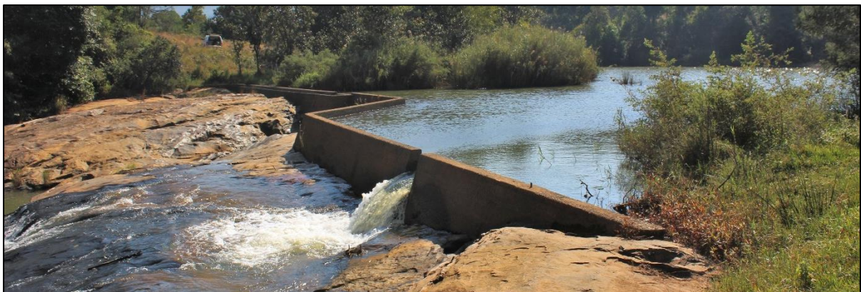
Figure 60: An impoundment located on the Lusushwana River (March 2019)
