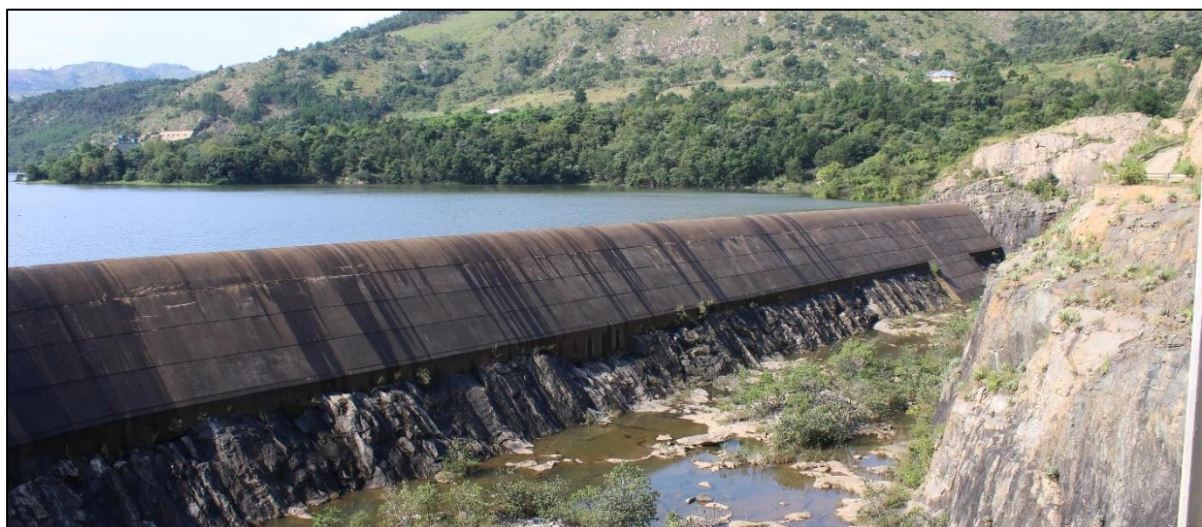
Figure 8: The Luphohlo Dam on the Lusushwana River upstream of the proposed impoundment (March 2019)
