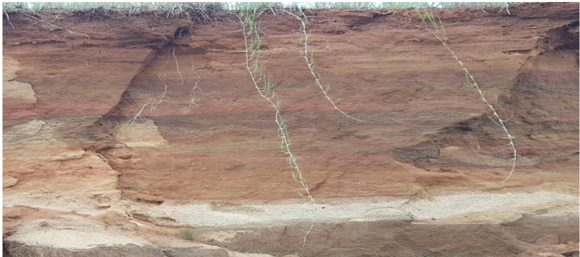
Photograph 3: Evidence of Leptosols found at the Nondvo Dam Site
