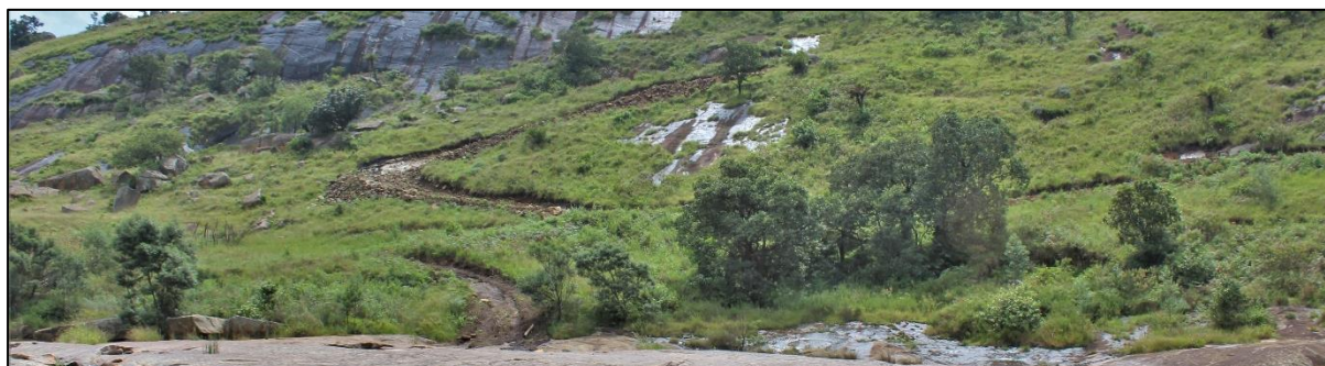
Figure 12: Geo-technical investigations at the proposed Nondvo Dam wall (March 2019)
