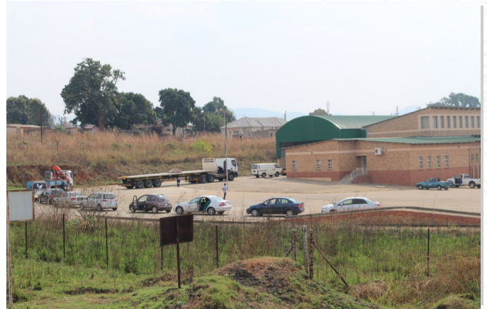
Test Station at Matsapha
