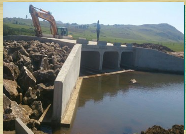
Construction of Hawane in-house bridge
