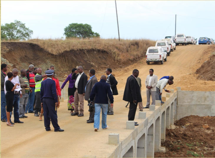
An in-house completed bridge at Mahlangatsha end of January 2015.
