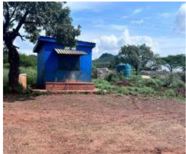
Figure 4-28: Water Kiosk at Esiphambanweni
