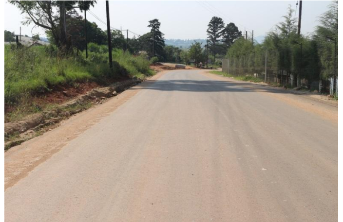
Njingeni – Malkerns Research Station road, which is nearing completion
